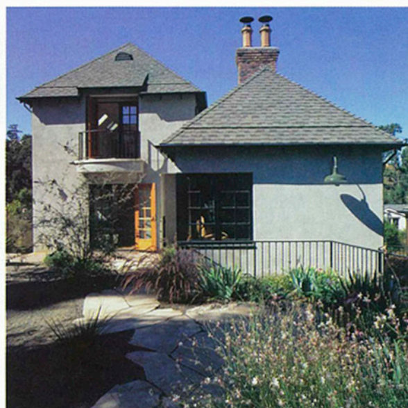
The roofs don't overpower the backyard. Notching the foundation into the hillside put the floor on the same level as the backyard. That decision, along with breaking the mass of the house into two roughly equal portions, reduced its bulk. Photo taken at D on floor plan.
