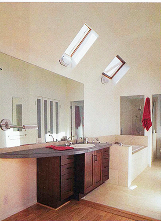
The bath is open to the bedroom. A mahogany cabinet topped with a curving concrete counter links the upstairs bedroom with the master bath. The shower walls, the tub surround and the bathroom floor are covered with limestone tile. Photo taken at F on floor plan.
